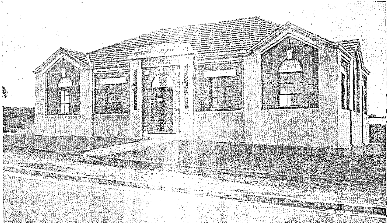
TOP PICTURE:—B.C.C. Substation seven-panel room and switchboard; 11,000-volt, 800-amp., 2,560,000 K.V.A.-rupturing capacity. BOTTOM PICTURE:—B.C.C. Substation containing 200 M.V.A. switchgear divided into two fireproof rooms
